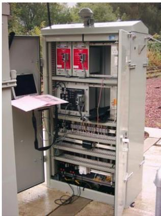
Figure 17 – Typical TRCM Installation
